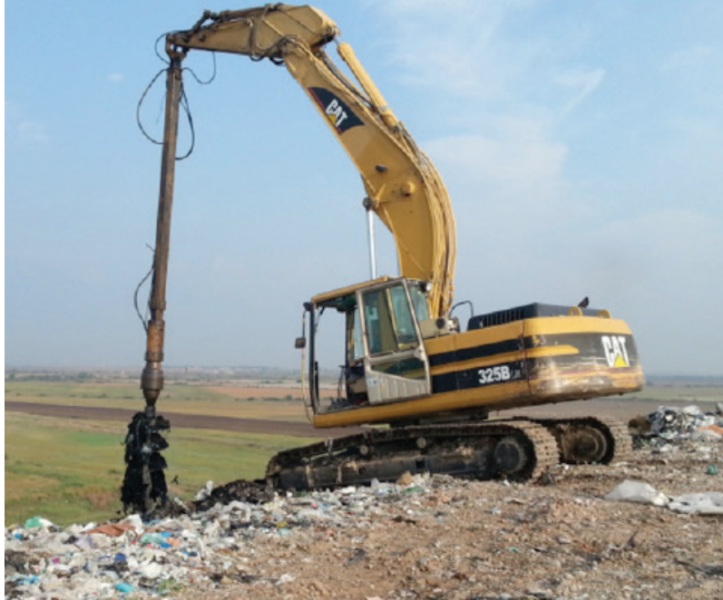
Drilling of degas wells, Arad, 2014.
